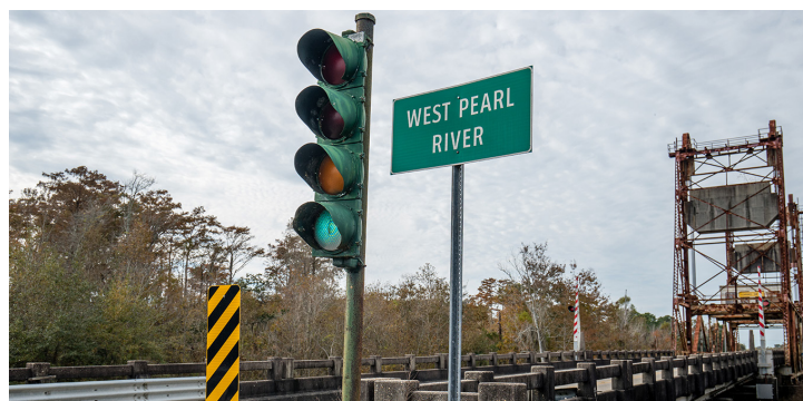
West Pearl River US 90 Bridge
