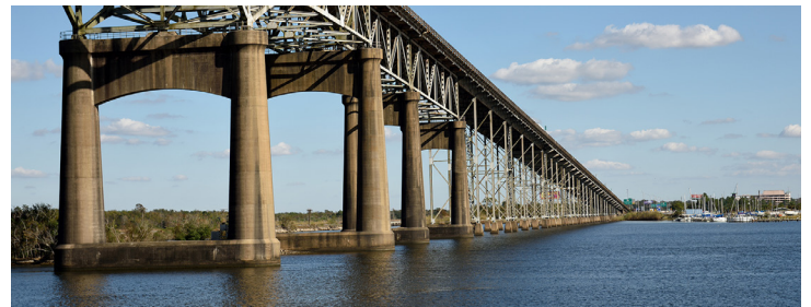
Calcasieu River World War II Memorial Bridge connecting Lake Charles and Westlake, Louisiana
