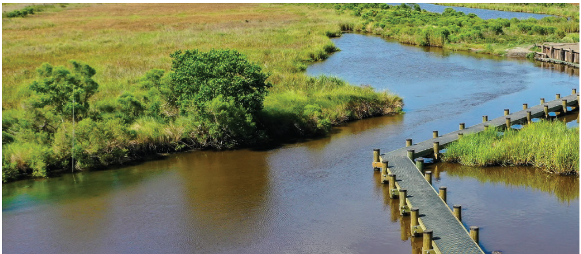
Examples of nature-based solutions in Louisiana. Starting from the top: restored floodplains slow and store floodwaters to reduce downstream flood risk. The middle image illustrates urban green infrastructure designed to temporarily retain stormwater during heavy rainfall, and the bottom image shows coastal wetland restoration that provides natural protection from flooding and storm surge while supporting wildlife habitat. Source: Louisiana Watershed Initiative.
