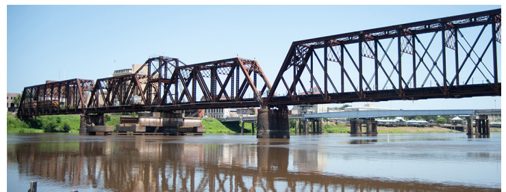
Steel railroad bridge in Monroe
