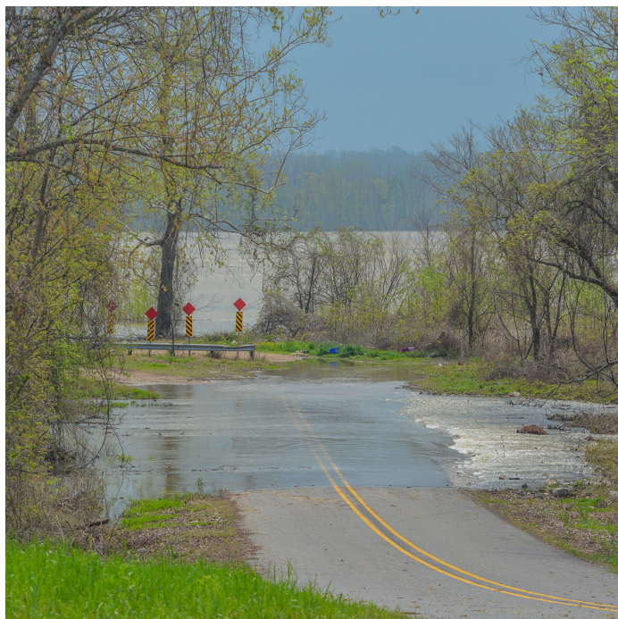
Tensas roadway flooding
