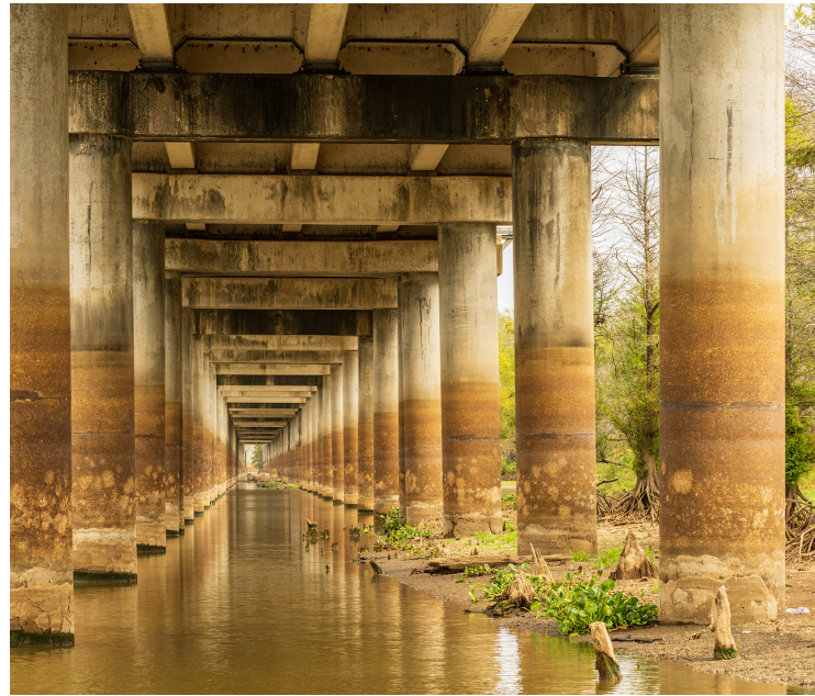
Pillars of the I 10 interstate bridge over the Atchafalaya basin near Baton Rouge, Louisiana
