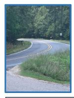
SKA's design team made a site visit to the LA 447 corridor, where it was observed that there are two (2) broken back horizontal curves south of Buddy Ellis Road near Bonnie Bleu Drive. Each have short tangents (~300'-400') between them with sharp curves having a radius appearing to be less than ~1000 feet. AASHTO states that, broken back curves should be avoided except where very unusual topo or right-of-way make them impractical.
