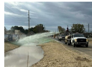
Figure 6: Re-Hydroseeding
