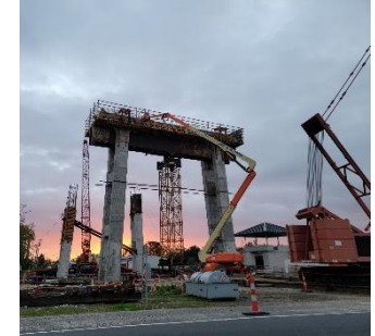
Figure 11: Moveable Bridge Construction
