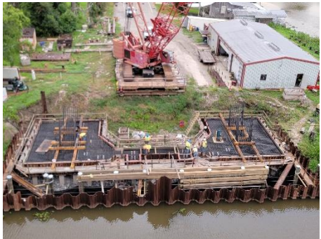
Figure 13: Foundation Steel
