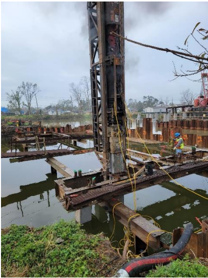
Figure 12: Pile Driving Operations
