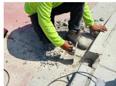
Figure 5: Repair of Deficiency
