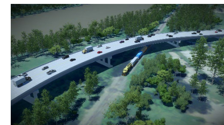
The new bridge will be 1,550' long and consist of a horizontally curved, haunched 4-span (185'-225'-300'-225') steel plate I-girder main span continuous unit over the Union Pacific Railroad with BT-72 prestressed concrete girder approach spans.
