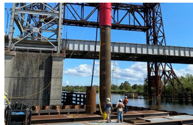
GeoEngineers oversaw the dynamic testing of a 48-inch diameter steel pipe pile for the new bridge's main pier.
