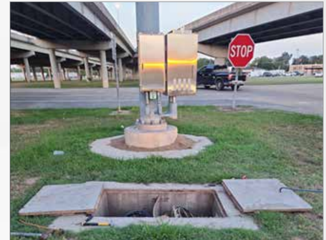
Existing ITS Site upgraded from wireless to fiber communications
