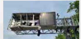
Damaged DMS sign inspected by team members before removal
