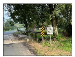
It is a three-span bridge with a precast concrete panel deck, a wide barrier curb walkway on both sides but no connecting sidewalks. It is supported on timber pile bents with timber caps, timber end bents and timber wingwalls. There is subsurface drainage in all four bridge quadrants:
