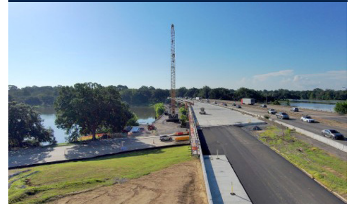
I-10 City Park Lake Bridge ongoing construction facing east above Dalrymple Drive
