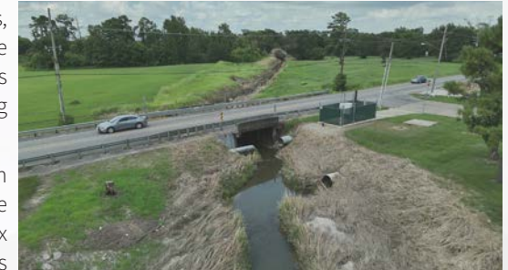
5. Figure 3: Bridge and Sewer Lift station near Pecan Acres Drive
