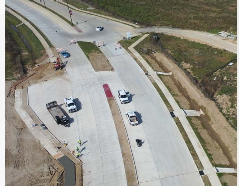
Aerial construction progress of the J-turn intersections from initial preparation through concrete pavement placement
