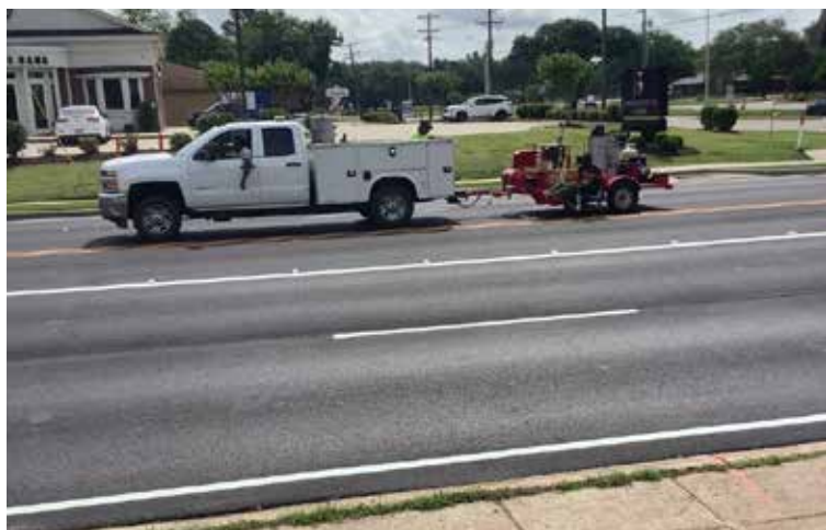
Pavement marker installation on LA 1 in Caddo Parish
