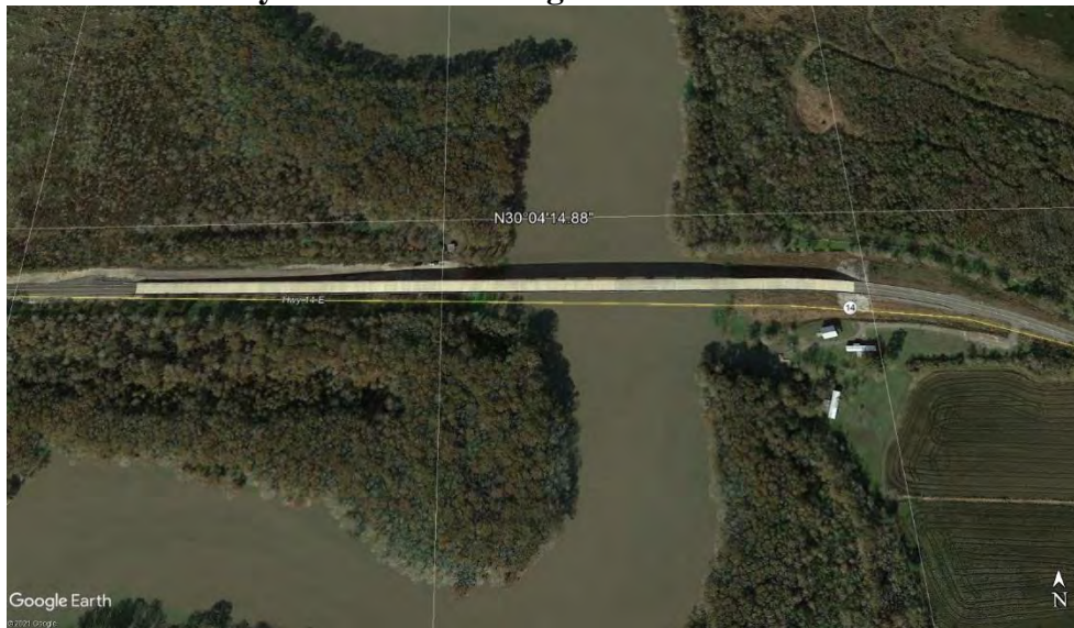
Bayou Lacassine Bridge
