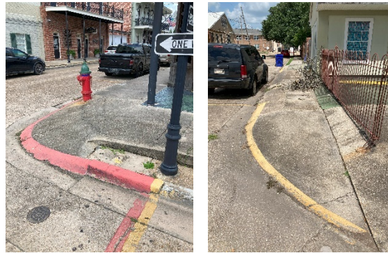
Figure 3: Curb Ramp Slope Issues
