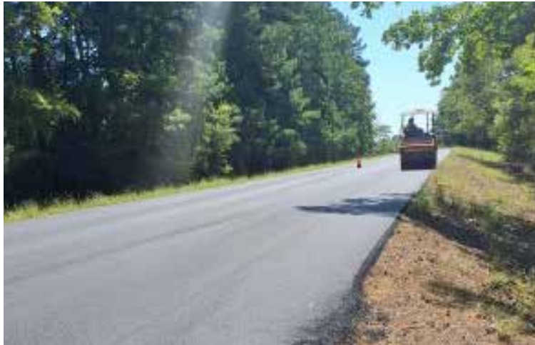
Finishing overlay on LA 9 in Bienville Parish
