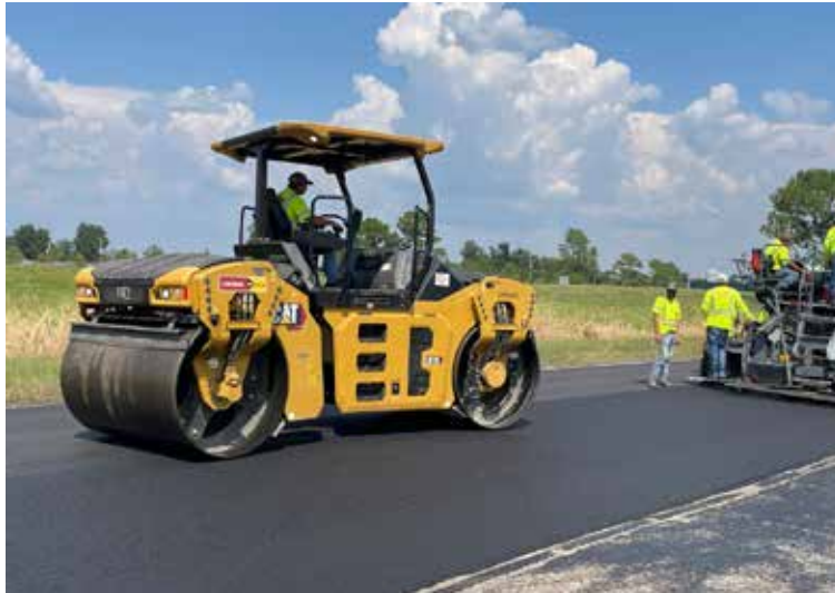
Asphalt crews in Calcasieu Parish
