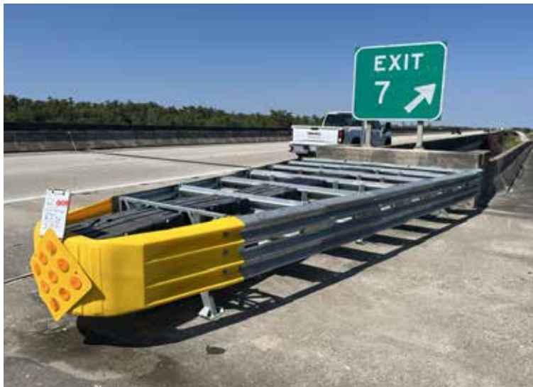
Guardrail repair on I 55 near Ruddock
