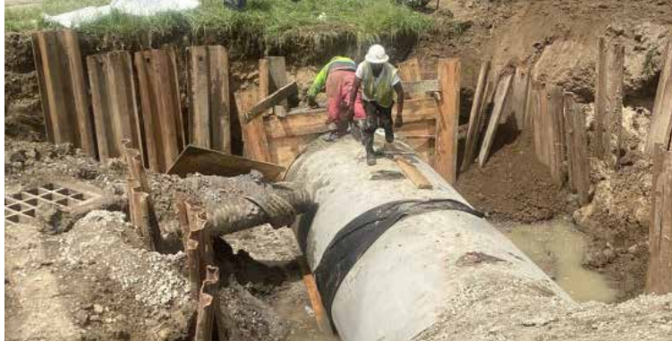
Pipe installation across LA 23 northbound near Empire
