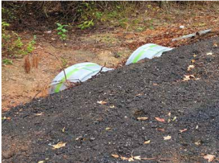
LA 834 cross drains in Morehouse Parish
