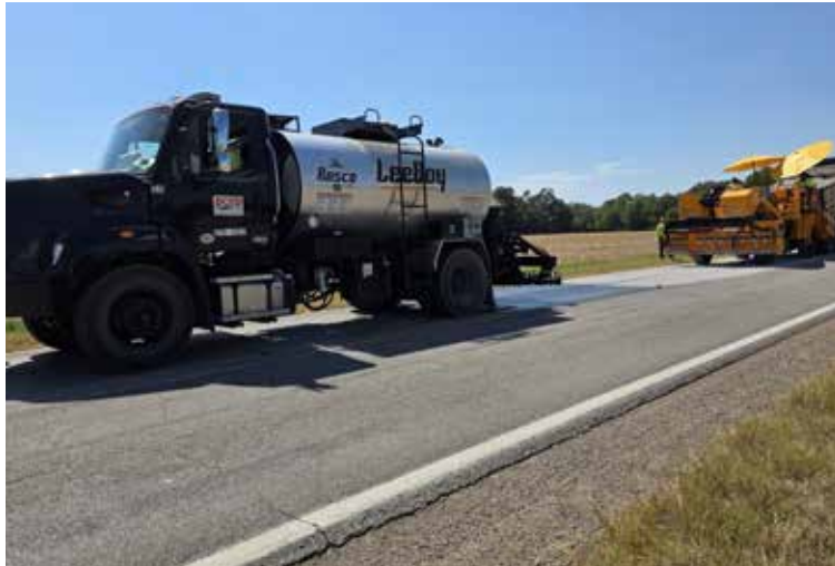
Crews applying chip seal to LA 130 in Franklin Parish
