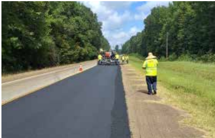
Overlay on U.S. 371 in Webster Parish
