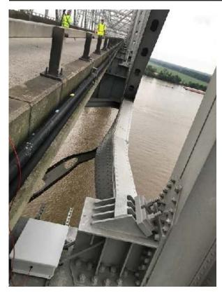
Following a bridge impact by a barge crane, the Sunshine Bridge was closed until emergency repairs could be completed. Modjeski & Masters was tasked with assessing the overall condition of bridge and design of repairs. BDI was subcontracted to assist in inspection and to provide instrumentation and structural monitoring.
