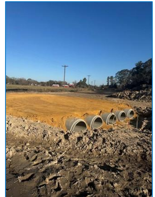
Culverts installed under McHugh Road
