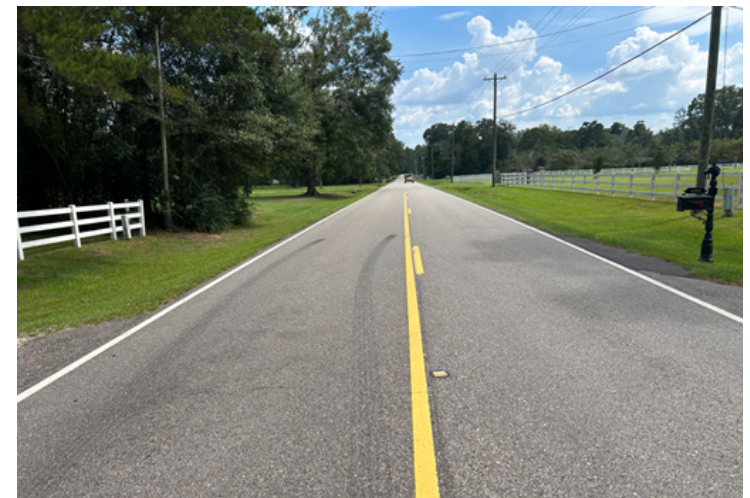
H.013546 Thibodeaux Road Improvements
