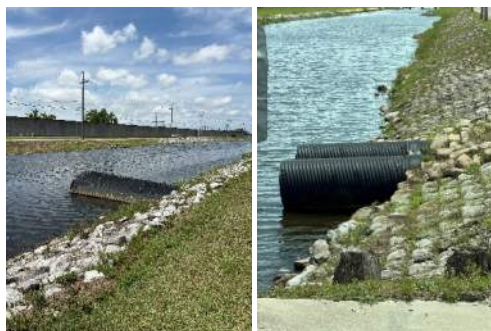
Figure 1: Drainage Lateral Connections
