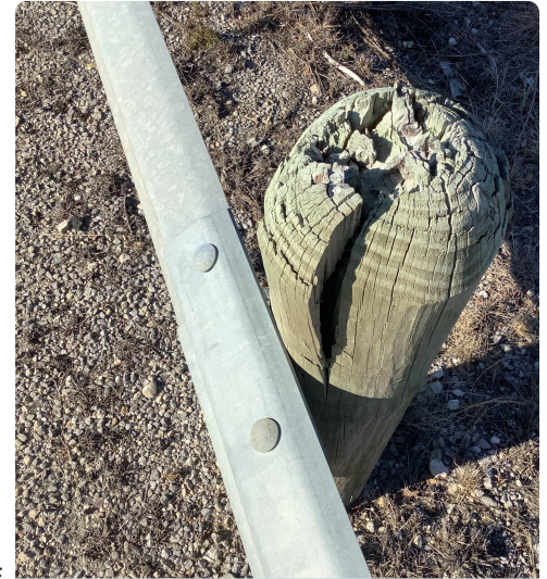
Existing guardrail and embankment condition will factor into methodology
