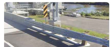
Typical LADOTD MASH Compliant Bridge Attachment
